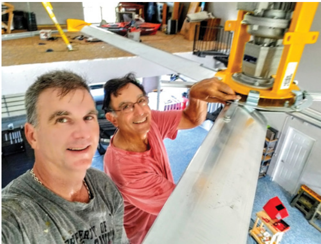
A Big Ass Fan with a 14-foot fan-blade diameter was chosen to provide cooling for the hangar. The fan motor's heavy weight required hoisting it into position with a Skyjack from below.
