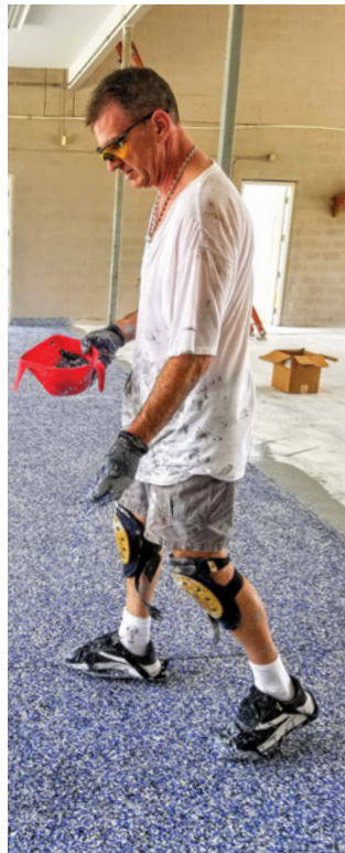
Berry apprenticed with with Tim McGill (and his family crew) at Distinctive Concrete Concepts and learned best practices for epoxy coating a floor for a huge wow-factor. Shown here are Berry, right and his father, Len, left, during the process.
