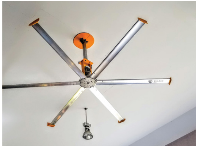
A Big Ass Fan with a 14-foot fan-blade diameter was chosen to provide cooling for the hangar. The fan motor's heavy weight required hoisting it into position with a Skyjack from below.
