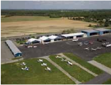
Summit Aviation's hangar complex in Middletown, Delaware.
