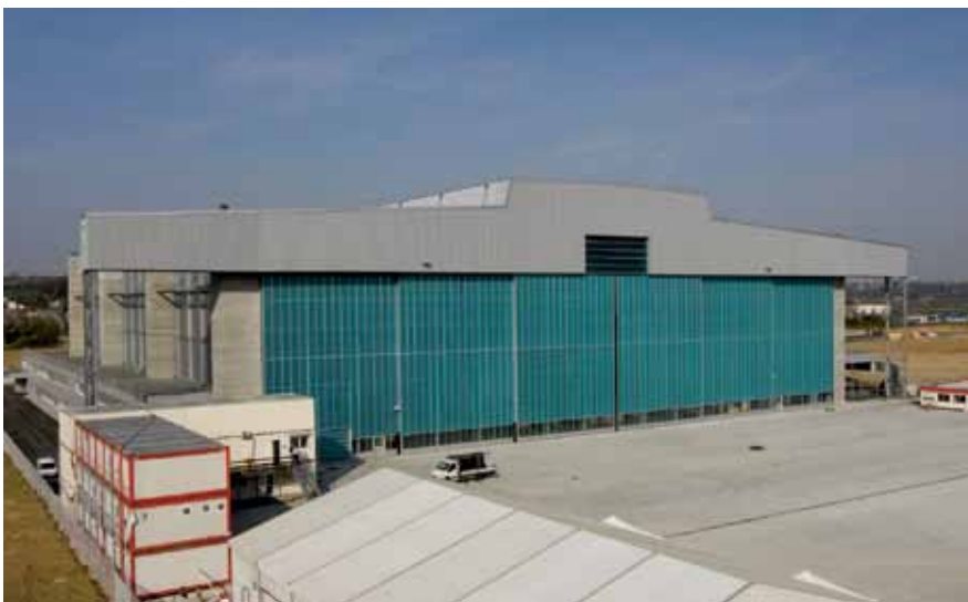
Jet Aviation Basel's new hangar has space to service an A380 and B747 at the same time.
