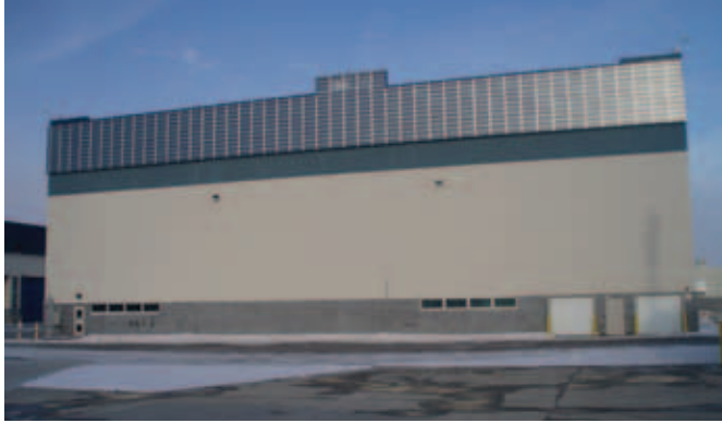
Left: Bombardier's plant engineering group authorized the recent installation of a Lubi, a wall-mounted solar air heater at its 40,000-square-foot research and development facility at the Mirabel Airport, Mirabel, Quebec. The solar collector manufactured by Enerconcept Technologies, Magog, Quebec, is amidst a two-year payback for that application. The 145-foot-wide x 12-foot-high Lubi aesthetically simulates architectural windows and covers about 25-percent of the 7,600-sq ft masonry wall. Right: Thermal imaging illustrates the dramatic rise of temperature in the solar collector versus ambient air and the building wall temperature below the Lubi. (Photos courtesy of Enerconcept Technologies) Right: Thermal imaging illustrates the dramatic rise of temperature in the solar collector versus ambient air and the building wall temperature below the Lubi™. (Photos courtesy of Enerconcept Technologies, Magog, Quebec)
