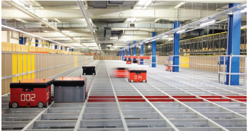
Lufthansa Technik installed AutoStore as part of a modernization program at their Hamburg locale.
