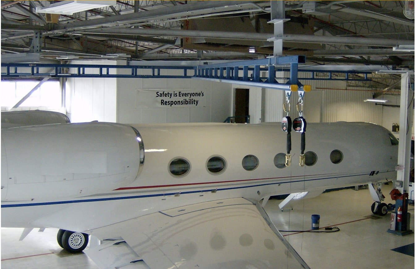
This low headroom hangar suits a system like the Gorbeltwo person Tether Track. Gorbeltwo image.
