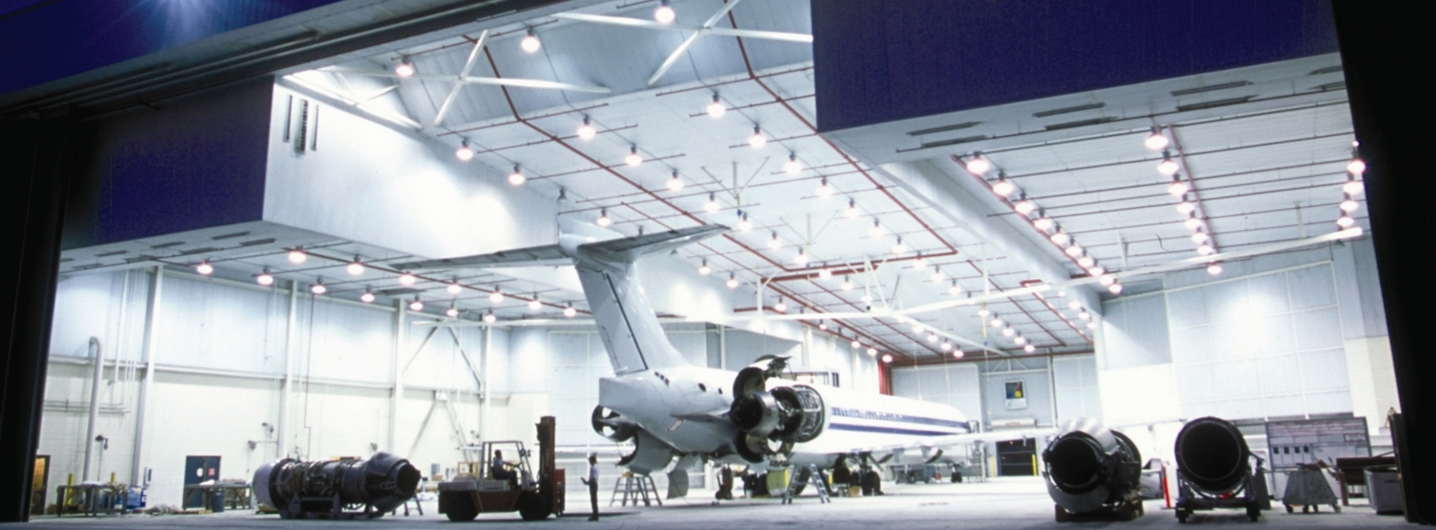
AAR Services' airframe MRO facility at Oklahoma City.
