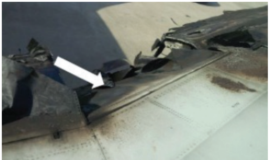
Graphic 2. Left wing and flaps that were severely burned from the fuel fire (NTSB Photo).
