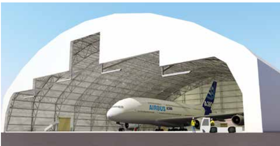
This A380 capable hangar, measuring 300ft by 300ft and 40ft high, is being supplied by Rubb Buildings to an undisclosed customer at an undisclosed location. Rubb Buildings image.
