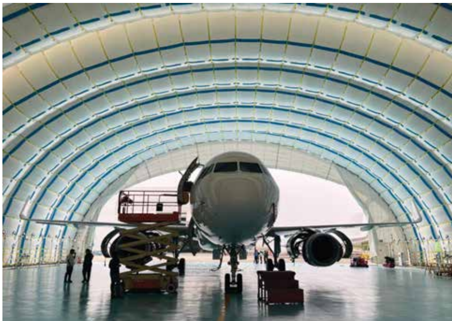
In May this year, GMR Aero Technic in Hyderabad, India, took delivery of this 45m wide Buildair hangar. Buildair image.
