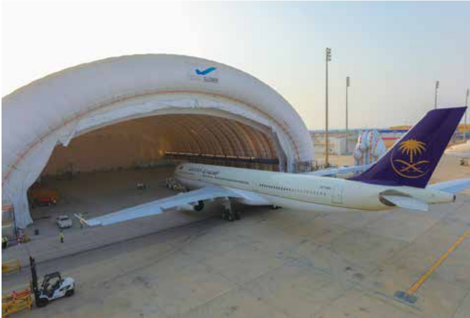
The world's largest inflatable building — a 75m wide hangar supplied by Buildair for Saudia Aerospace Engineering Industries in Jeddah. Buildair image.
