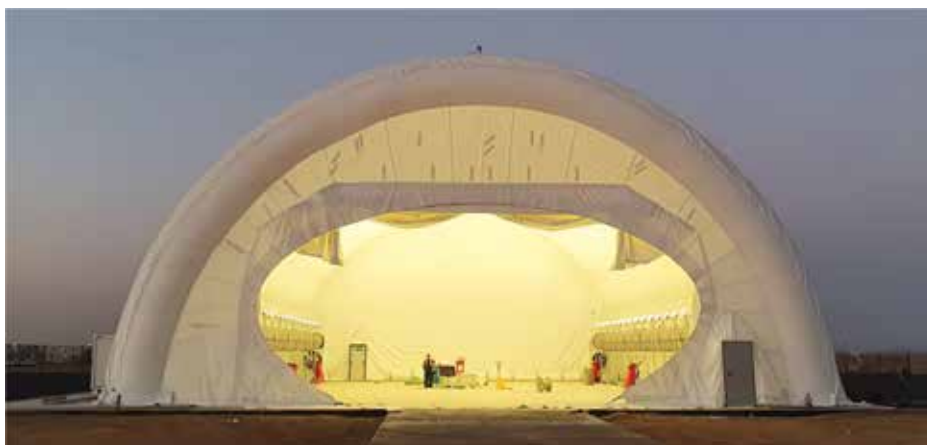
Buildair's latest project is a hangar for The Helicopter Company of Saudi Arabia in Jeddah. Buildair image.
