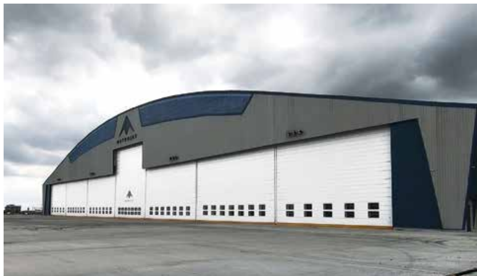
This maintenance hangar for Hong Kong-based Metrojet at Clark in the Philippines has five vertical lift Champion doors. Champion Door image.
