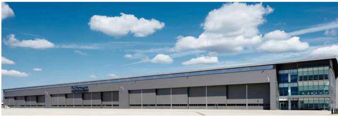
Jewers Esavian Type 126 doors are fitted to the Gulfstream Aerospace Corporation Customer Support Service Centre at Farnborough Airport in the UK. Jewers Doors image.
