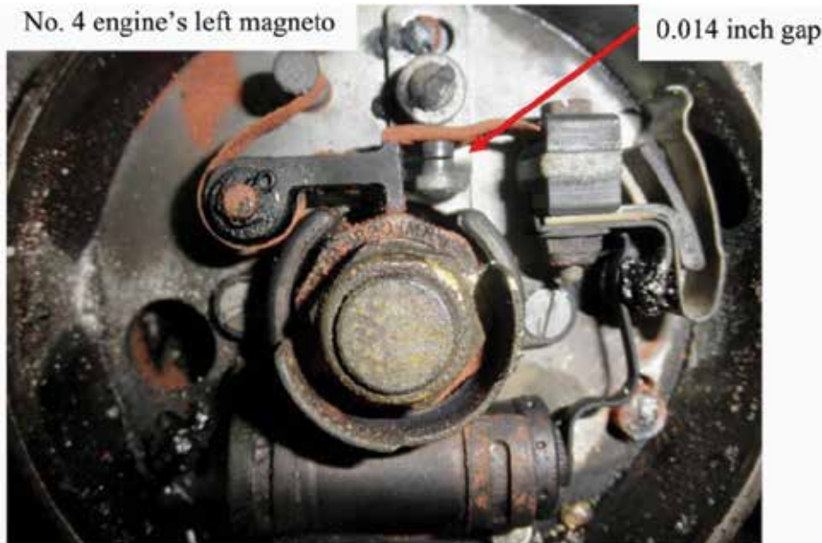
Photo 11: Close-up of the No. 4 engine's right magneto, showing the improper gap between the points.
