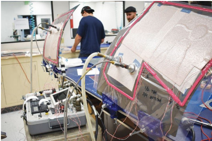
Bag (a vacuum bag) and bonder (a hot bonder device) are components of a hot bonding process, where the vacuum bag seals the repair area, and the hot bonder applies precise heat and vacuum to cure adhesive or resin, ensuring proper compaction, bond strength and restoration of structural integrity to the composite structure. Abaris image.
